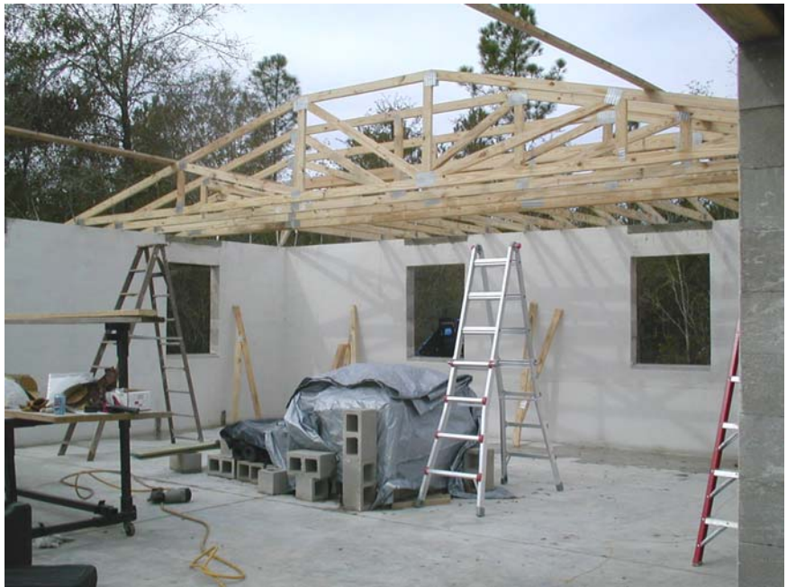
Figure 52. Roof trusses being installed.
