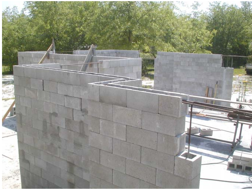
Figure 39. Corner blocks and linear half blocks.
